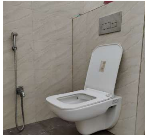
Disabled Friendly Washroom
